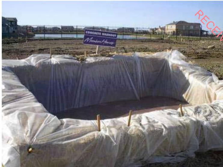
**Plate 2.3: Typical Temporary Concrete Washout Area**
